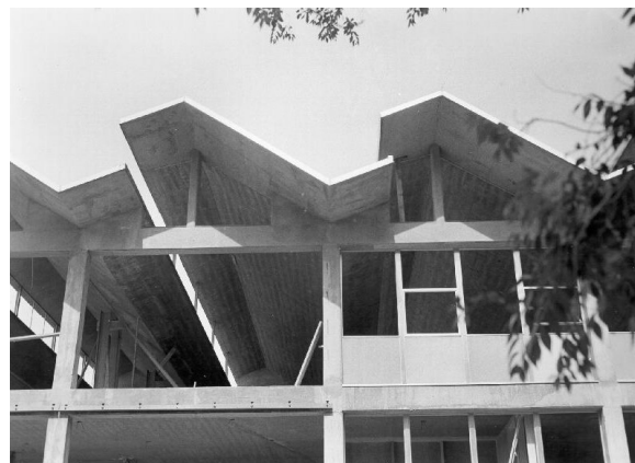
Figure 8: simple folded plate roof, providing increased bending stiffness.
